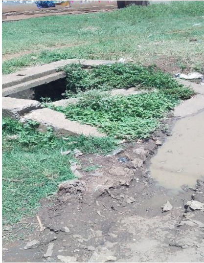
Plates 10: Damaged sewer manhole in Mjini
