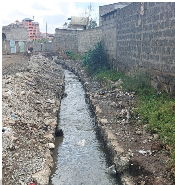
Figure 41 - Existing Drainage System in the Settlement
