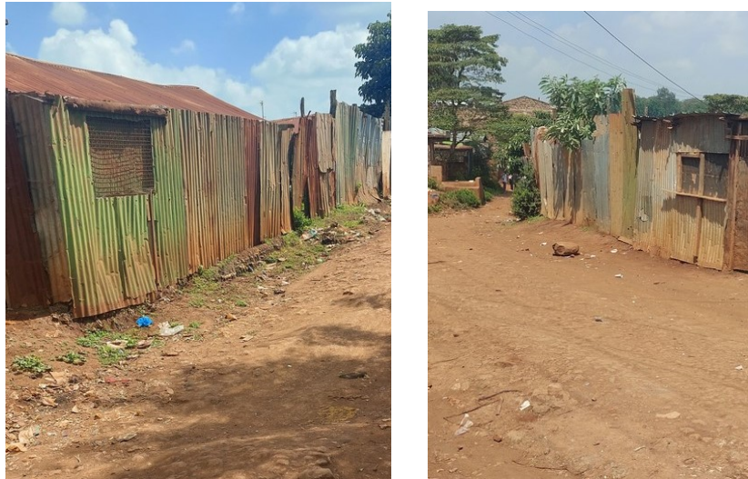
Figure 27 – Typical Types of Existing Houses in the Settlement
