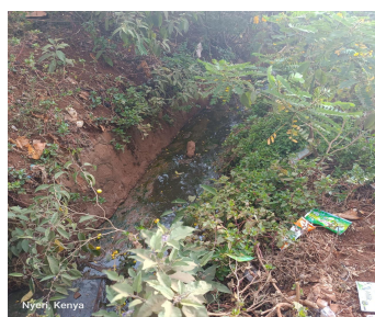
Figure 2- 1: Sewer flows in pre-existing storm drains
