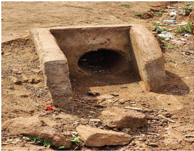
Figure 2- 1: Existing concrete pipe culverts.
