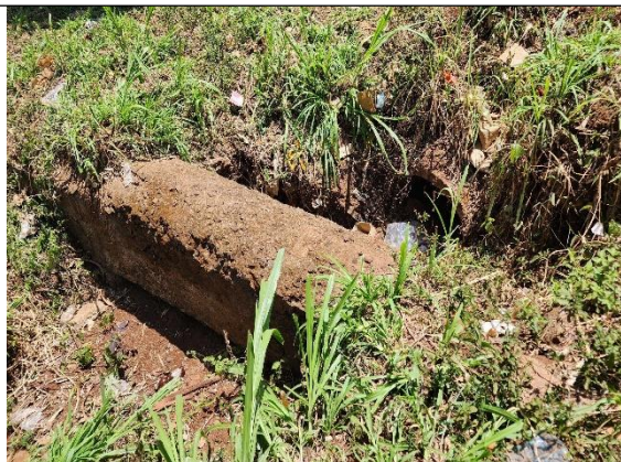
A Cross Pipe Culvert With Outlet Partially Obstructed By A Sewer Concrete Pipe
