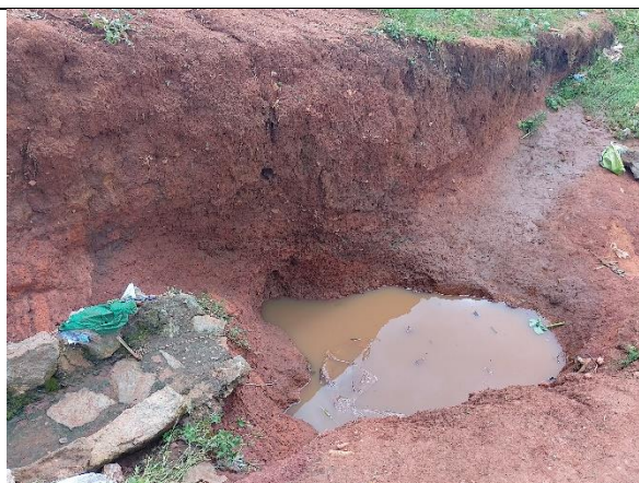
Plates 14: Eroded drainage in Tuwani
