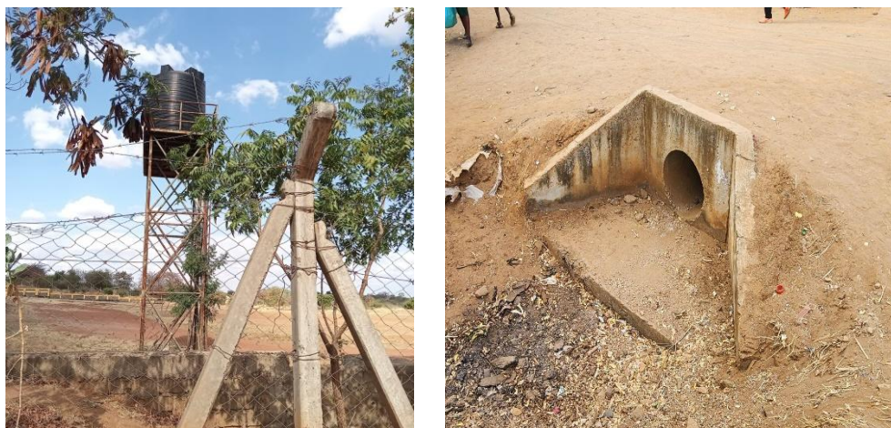
2No 5000-Litre water tanks at Marimanti Stadium Existing concrete pipe culverts
