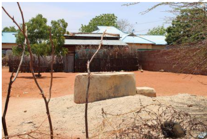
Figure 4-4: Shallow well with a raised well head
