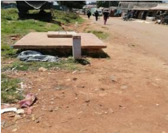
water chamber and marker post for the water pipeline within the settlement
