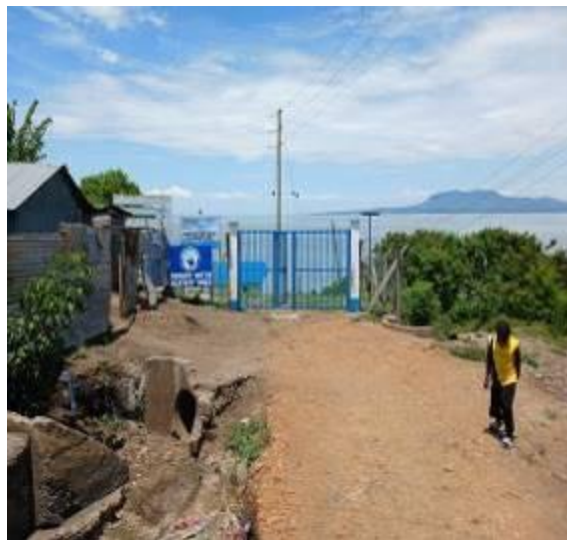
Water Treatment Plant in the area
